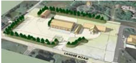
and sided building. This is a very efficient plan which satisfies the needs of the Village. The new building will include vehicle storage, mechanics bay with lift stations, wash bay and parts storage. The site work includes concrete aprons in the front and rear of the building and in front of the salt storage building.
